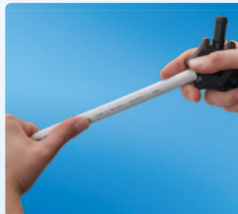
2. Bevel the pipe until a small chamfer is visible
